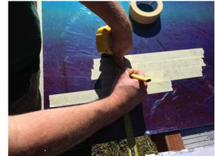
**Step 4: CUTTING** - Double check all measurements before starting to cut the splashback. Use a circular saw for long cuts and a jigsaw for more detailed cut-outs.
